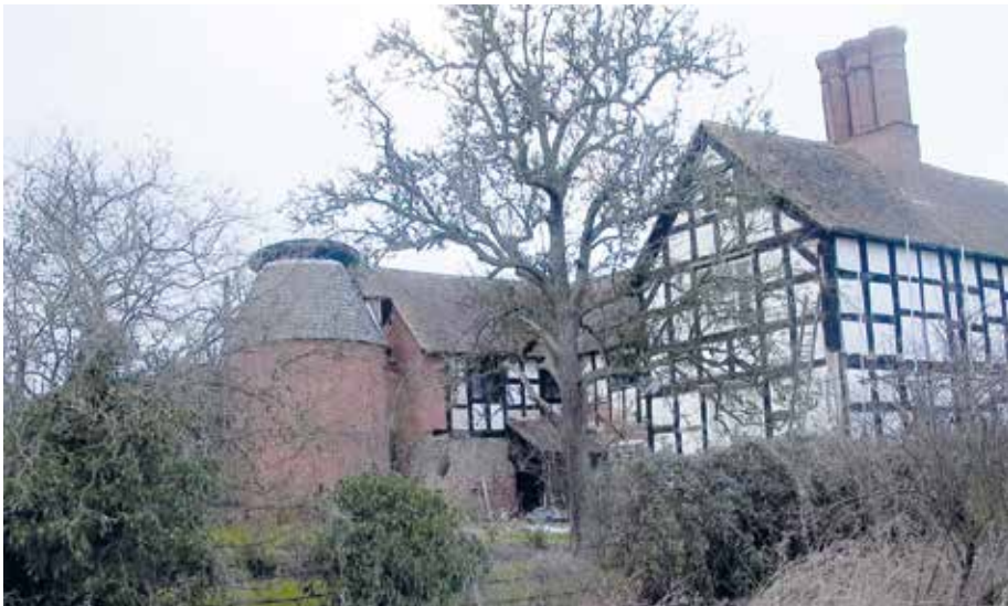
Back of Walsopthorne farm showing a hop kiln. "the Crops of Hops (in the two years) were so deficient as scarcely to be sufficient for payment of Parish rates and Taxes leaving the Planters at the loss of the Greater Part of the Rent, Tithes, Labour and Interest of Capital." Petition to the Treasury by 500 farmers in 1831. Signatories included Stephen Pitt of Walsopthorne
