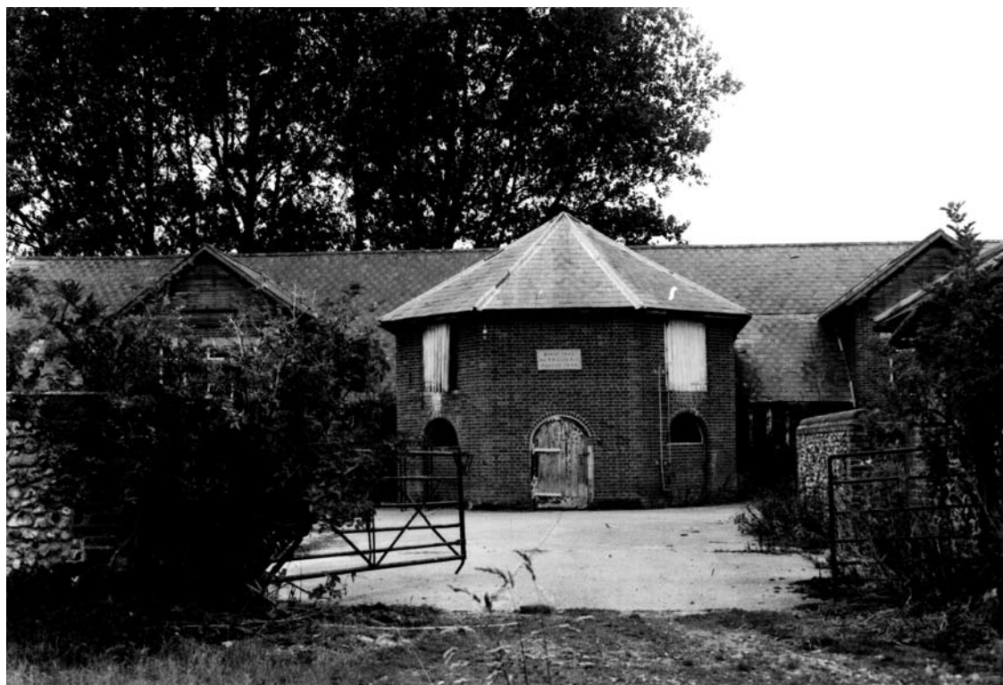
Wheel houses are rare in Suffolk where a surplus labour force meant there was little incentive to abandon threshing by hand. The plaque on this example at Grange Farm Hengrave states that the building was burnt down (presumably by incendiaries) in 1848, but rebuilt by Sir T.R.Gage in 1849.
