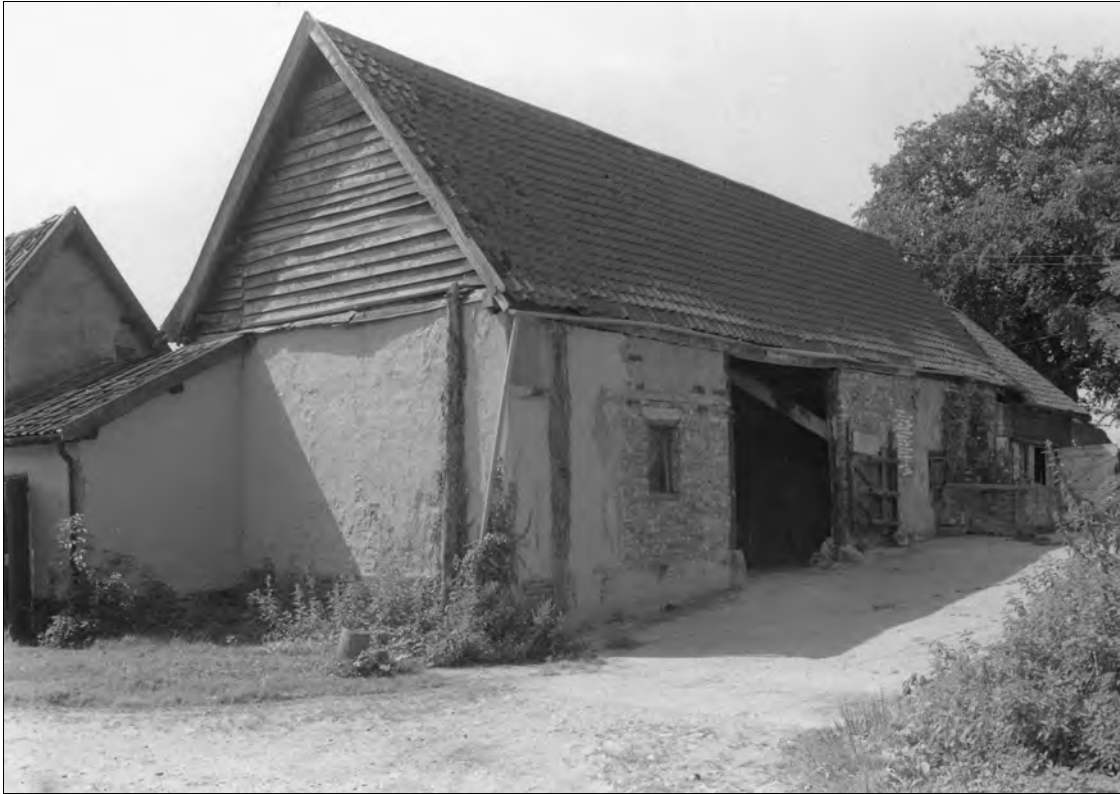
11. A seventeenth-century timber-framed barn at Church Farm, Hethel, Norfolk.
