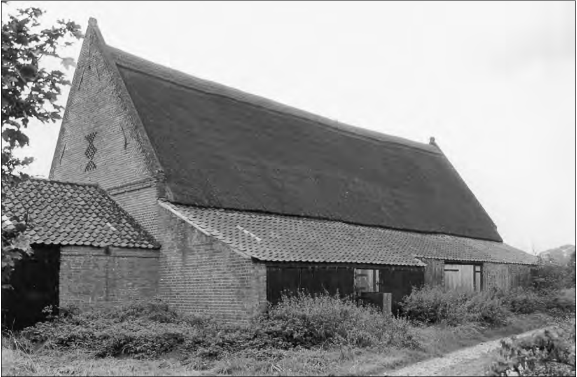
9. An early eighteenth-century barn at South Burlingham, Norfolk.
