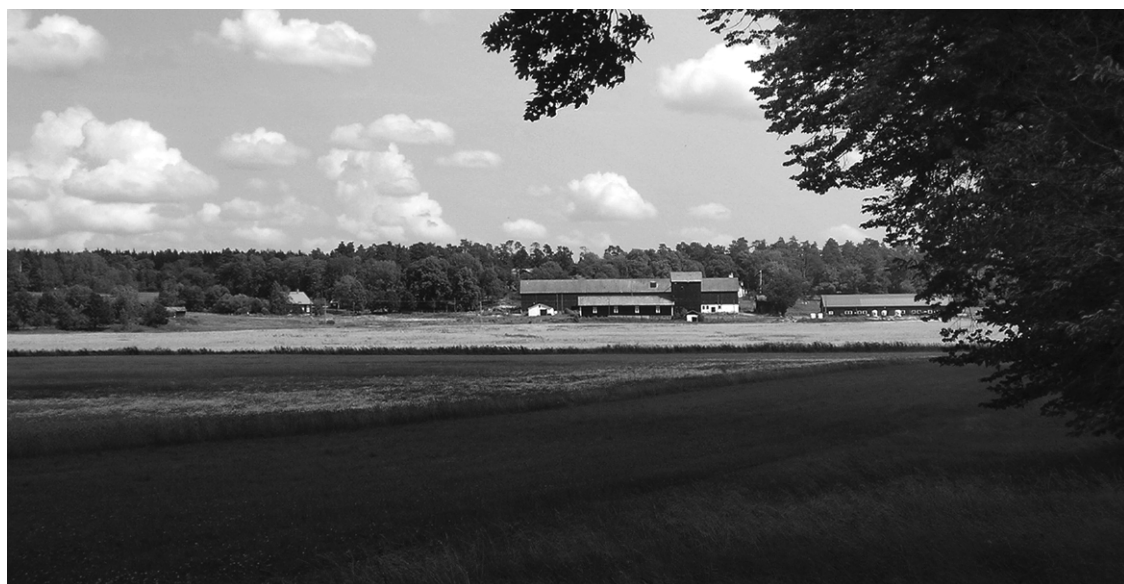
FIGURE 3. Farm buildings at Krusenberg including the old cowshed (white walls) where dairy production took place from the 1870s to the late twentieth century. Photo: Carin Martiin, 2008.
